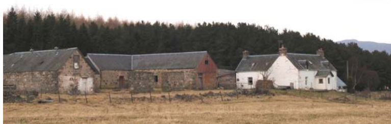
Fig. 5 : Existing U shaped steading
